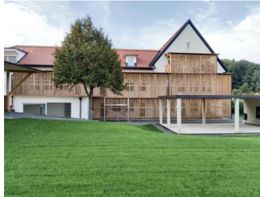
Climate-fit renovation of the primary school
