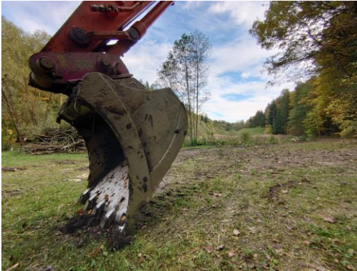
Safety measures at the retention basin
